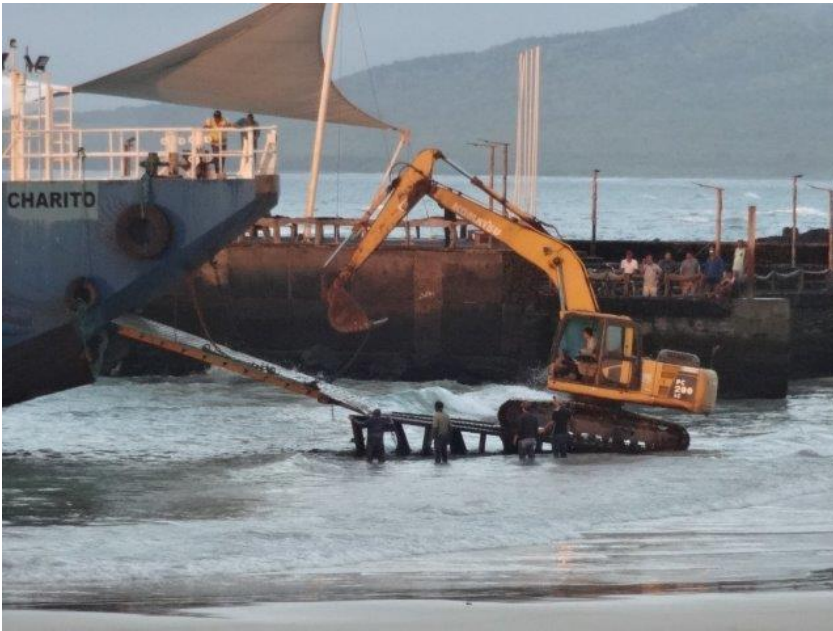
Plate 8: Construction on Isabela requires an ancient approach to plant delivery!
